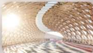
Atyrau Bridge Astana
